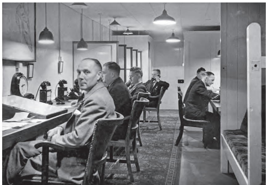
Southampton Docks Control Room
